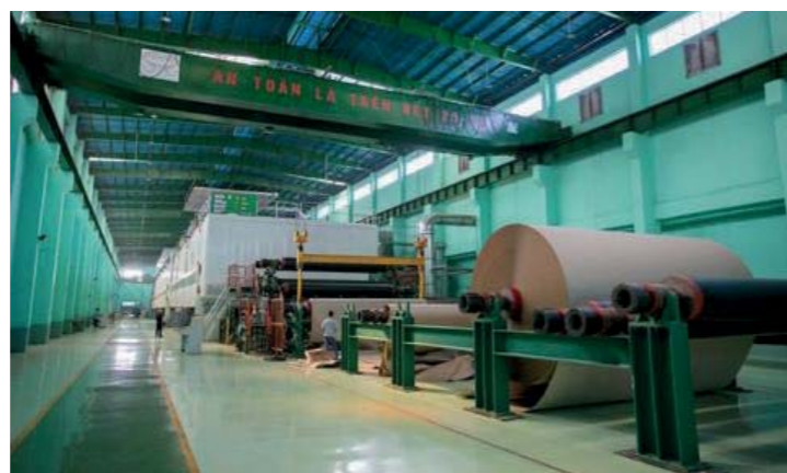
Dohaco's latest board paper machine is operated by ABB's electrification and automation system
