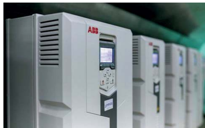
ABB's multi-drives and single drives at work in the mill
